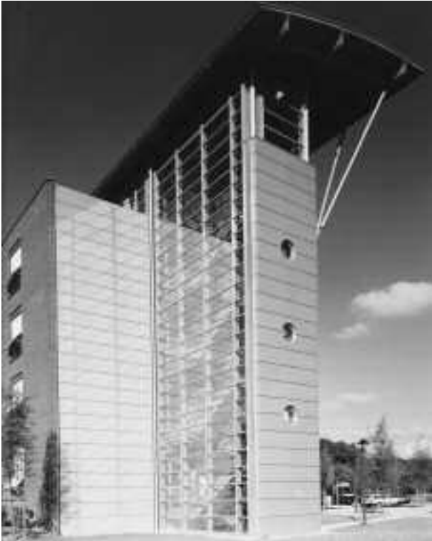
Decorative and functional: Combination of lustrous silvery aluminium façade panel faces and window profiles at the employment exchange in Bremerhaven
